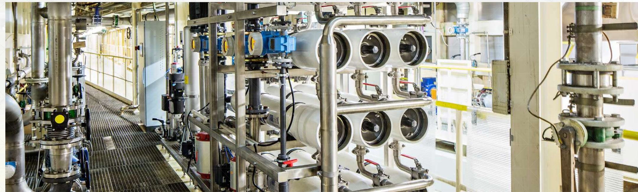
Reverse osmosis for production of demineralised water from vehicle body rinsing in the paint shop
